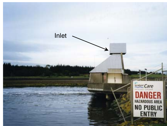
Inlet attached to building roof.
